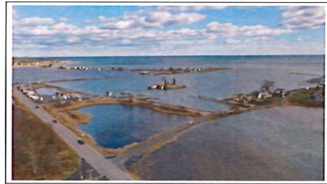
The picture above was taken at approximately 12:30pm on November 17, 2020. This was a 12.1 ft Spring or "King" tide. Note the "pond" in the center of the lot that enters the facility from the drainage swale located in the middle of the seawall. The next Spring tide will occur on Monday, January 23, 2023, where Rye Harbor will see a 13.06' tide.
