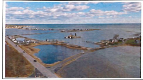
The picture above was taken at approximately 12:30pm on November 17, 2020. This was a 12.1 ft Spring or "King" tide. Note the "pond" in the center of the lot that enters the facility from the drainage swale located in the middle of the seawall. The next Spring tide will occur on Monday, January 23, 2023, where Rye Harbor will see a 13.06' tide.
