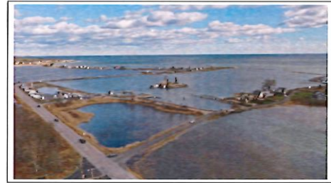
The picture above was taken at approximately 12:30pm on November 17, 2020. This was a 12.1 ft Spring or "King" tide. Note the "pond" in the center of the lot that enters the facility from the drainage swale located in the middle of the seawall! The next Spring tide will occur on Monday, January 23, 2023, where Rye Harbor will see a 13.06' tide.
