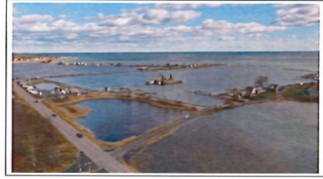
The picture above was taken at approximately 12:30pm on November 17, 2020. This was a 12.1 ft Spring or "King" tide. Note the "pond" in the center of the lot that enters the facility from the drainage swale located in the middle of the seawall. The next Spring tide will occur on Monday, January 23, 2023, where Rye Harbor will see a 13.05' tide.
