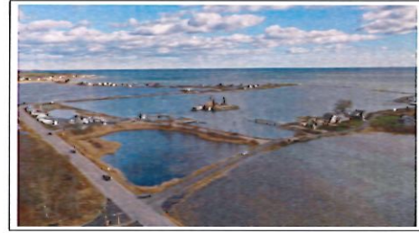
The picture above was taken at approximately 12:30pm on November 17, 2020. This was a 12.1 ft Spring or "King" tide. Note the "pond" in the center of the lot that enters the facility from the drainage swale located in the middle of the seawall. The next Spring tide will occur on Monday, January 23, 2023, where Rye Harbor will see a 13.06' tide.
