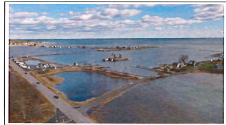
The picture above was taken at approximately 12:30pm on November 17, 2020. This was a 12.1 ft Spring or "King" tide. Note the "pond" in the center of the lot that enters the facility from the drainage swale located in the middle of the seawall. The next Spring tide will occur on Monday, January 23, 2023, where Rye Harbor will see a 13.06' tide.
