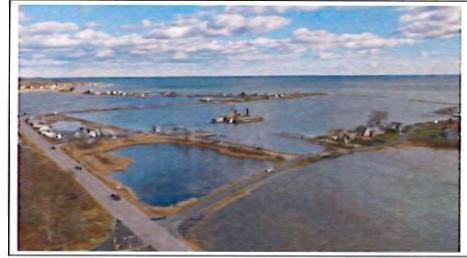
The picture above was taken at approximately 12:30pm on November 17, 2020. This was a 12.1 ft Spring or "King" tide. Note the "pond" in the center of the lot that enters the facility from the drainage swale located in the middle of the seawall. The next Spring tide will occur on Monday, January 23, 2023, where Rye Harbor will see a 13.05' tide.
